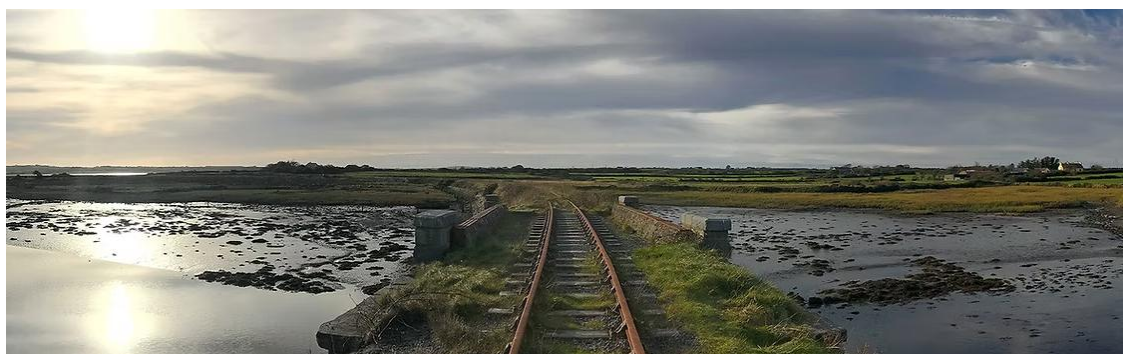
Figure 4-14 Existing Railway Bridge at Moyasta looking west
