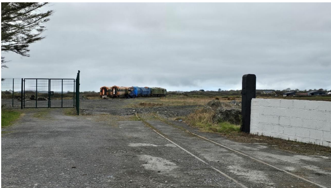
Figure 4-16 Existing tracks along the former railway line along which the proposed greenway will run on the approach to Moyasta village
