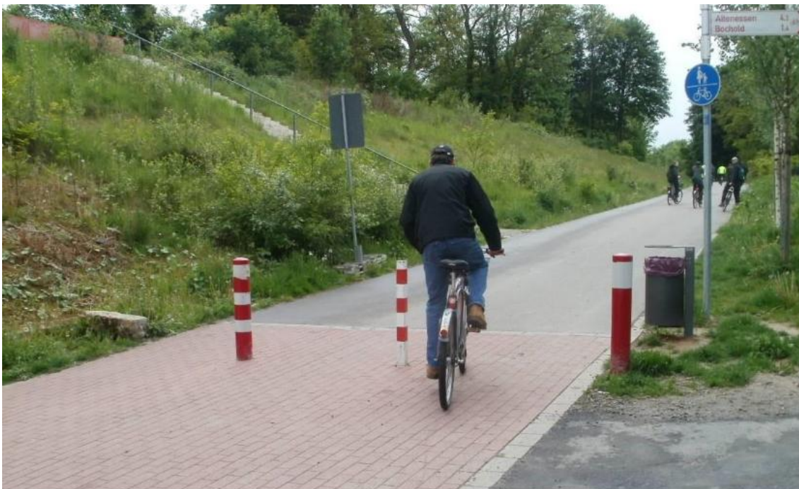
Figure 4-35 Simple Bollard Access - Generous width (Essen, Germany)
