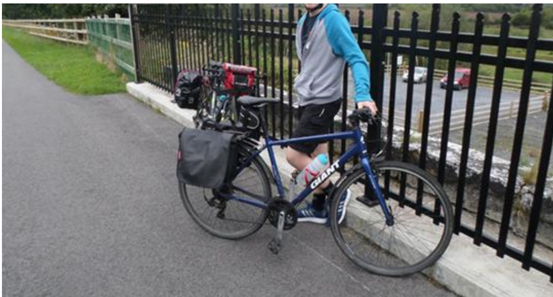
Figure 4-49 Example of a parapet/fencing (Location: Railway bridge on the Old Rail Trail between Athlone and Mullingar)
