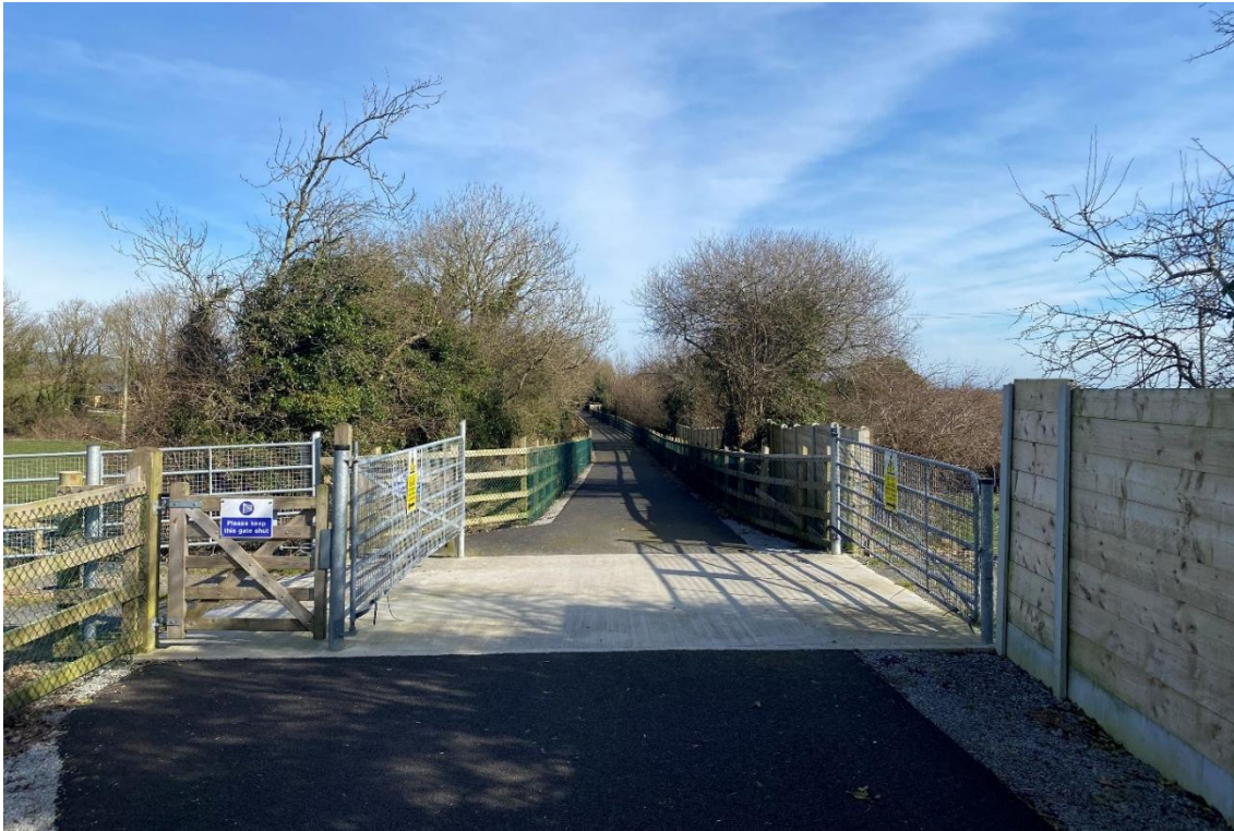
Figure 4-46 Example of enhanced farm crossing (Location: The Waterford Greenway)
